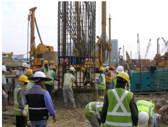
Test pile depths ranged from 69.5 m to 82.5 m on 1800 mm diameter to 3000 mm diameter rotary bored piles and 2800 mm x 1000 mm for the barrette.
