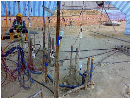
Even though concrete was only cast to cut off level, the reinforcing cage and O-cell related instrumentation was brought to platform level so that testing could be conducted from the existing platform level.
