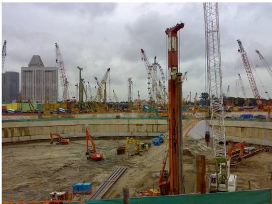
Design cut off levels across the site ranged from 13.0 m to 25.5 m below platform level and working pile tests had to be carried out before the excavation was started. Concreting of the piles and barrette was carried out to cut off level with the empty excavated bore carefully backfilled with clean sand fill material to platform level to maintain bore wall stability and for safety reasons.
